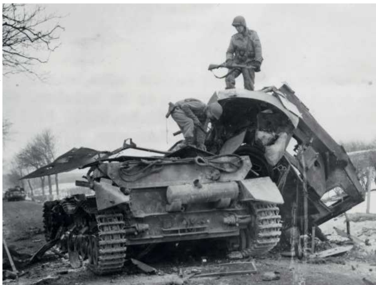
■ Right: GIs examine a destroyed Panzer IV Ausf. J. Against side hits, the 30mm armour could not withstand any Allied tank gun.
