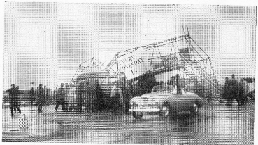
DISASTER: The chaotic scene in the straight, when a van struck the footbridge causing its collapse and the premature end to the meeting.
