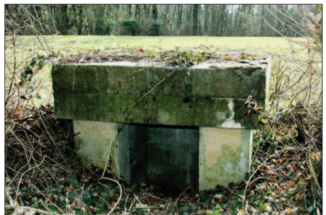
In many places near the 'W 2' compound — such as at Laffaux, Neuville and Vauxaillon — the Germans used ancient underground quarries to store equipment, supplies and food. They concreted the entrance for some distance, and sometimes installed Decauville narrow railway tracks to service the interior. Above: This is one of the three ventilation and escape exits built by the Germans for the quarry at Vauxaillon.
