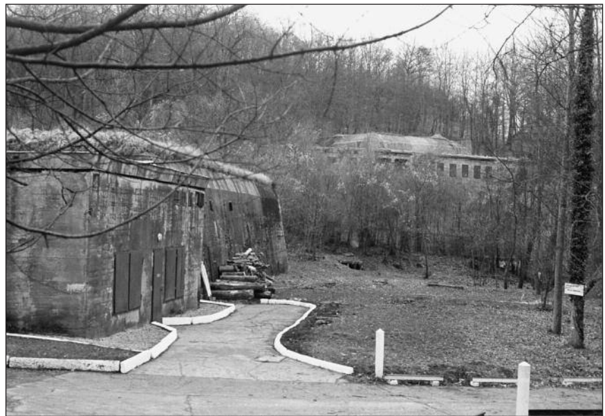
Another shot taken at the time of the CEC in 1982, this one showing a well-maintained Bau 4, which was a heavy bunker of the 'Baustärke A' type, that during the war had housed the FHQu teleprinter exchange. Note that its 'Vorbau' (annex) was built on one side only. In the background, across the railway line, stands Bau 1. The original German concrete road was still in perfect condition.
