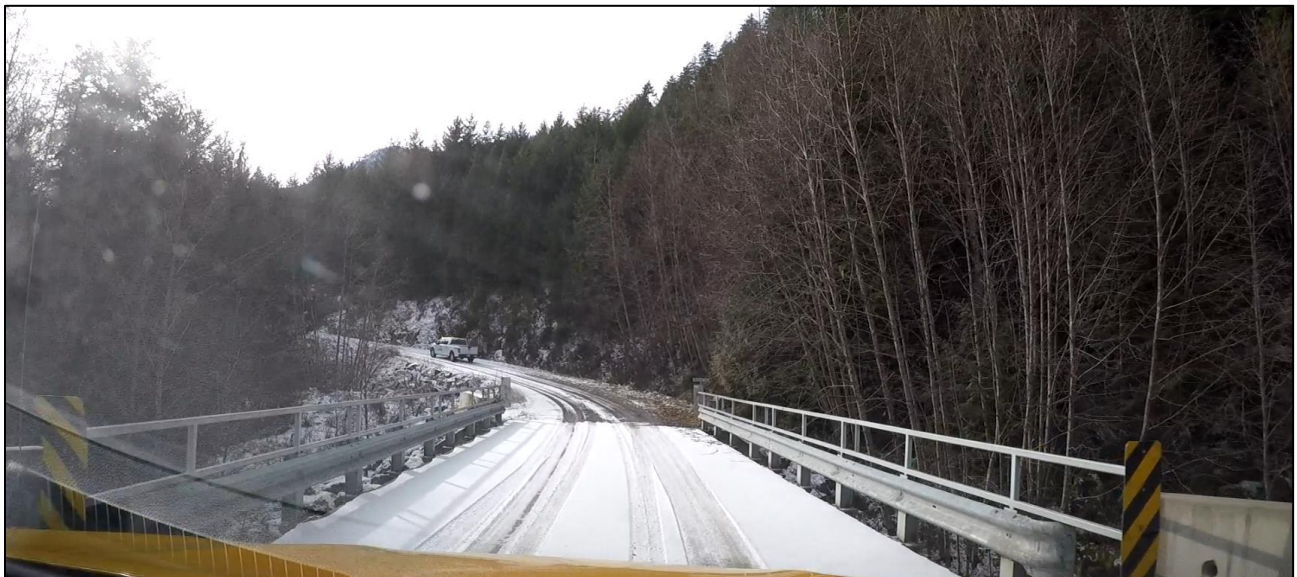
Figure 4.5: Bridge Structure Overtop of Watercourse that Feeds Sooke Lake Reservoir
