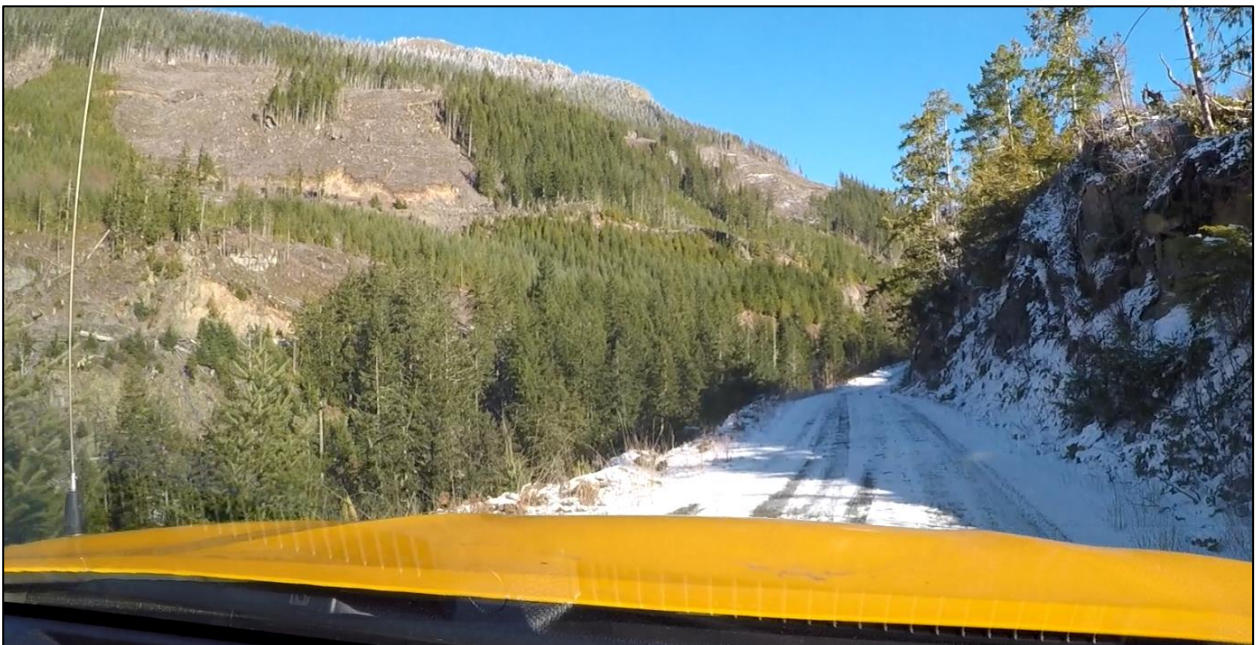
Figure 4.20: Old Renfrew Road Pinch Point between Steep Slope and Cliff-face
