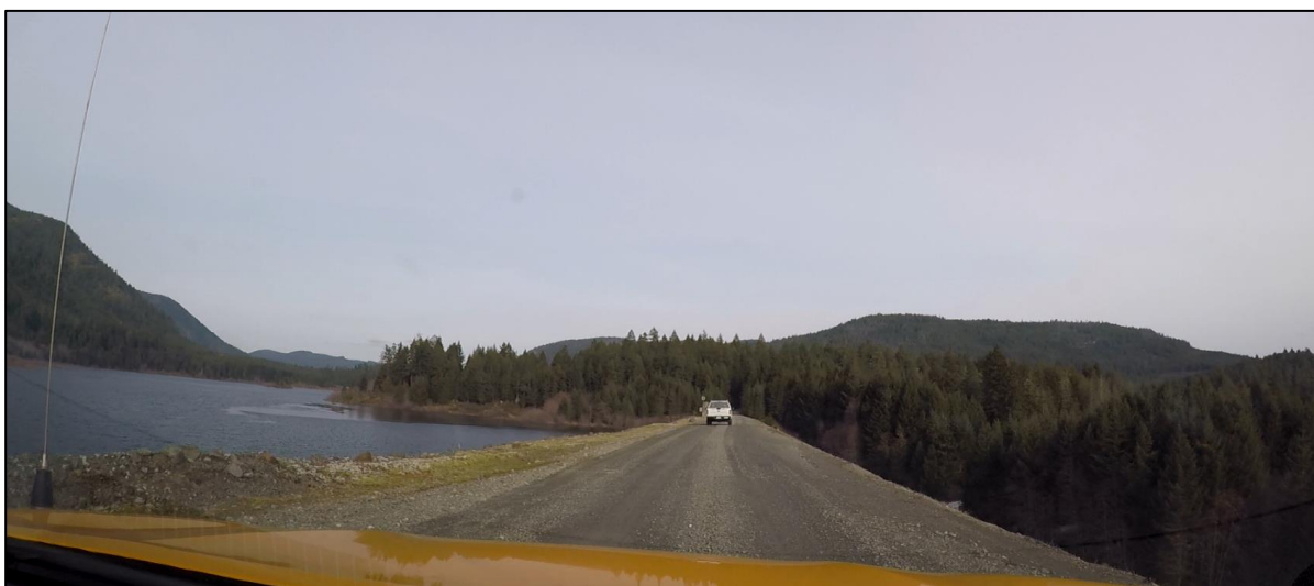
Figure 4.4: Causeway of Deception Reservoir Dam
