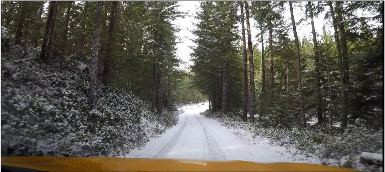
Figure 4.12: Example of Cross Section with Moderate Slopes on Niagara Main inside Watershed
