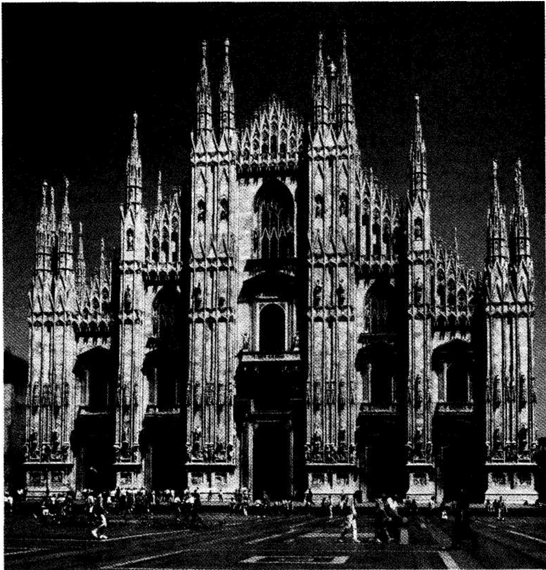
1-1. The west facade (main entrance) of Milan Cathedral, built in baroque style in the 16th century, with a retro-gothic third tier added later.
