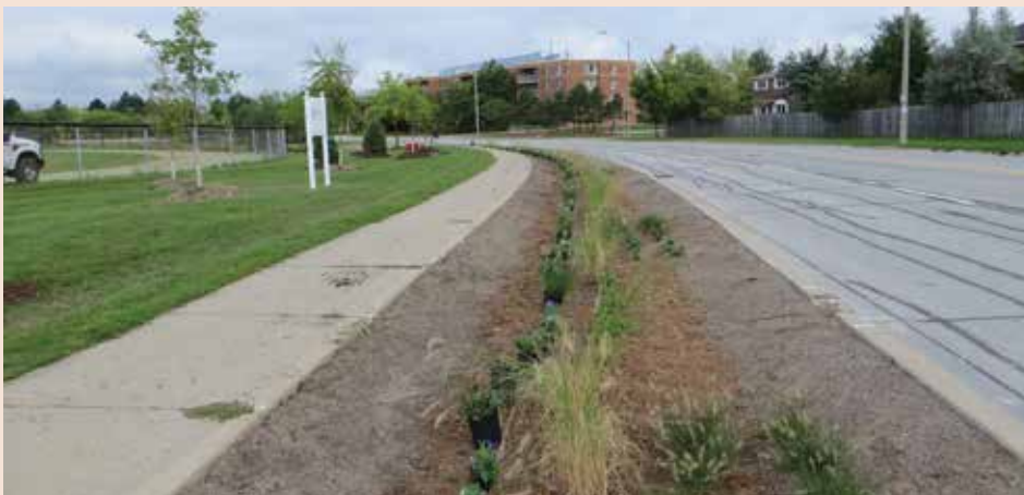
Bio-filter swales absorb and clean stormwater before it enters a local creek in Brampton, Ontario.
