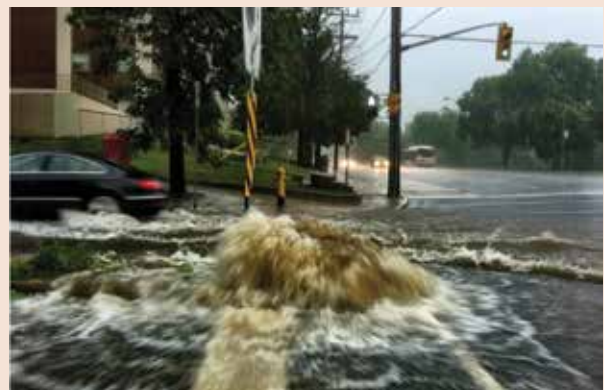
Photo credit: Toronto Hydro.
