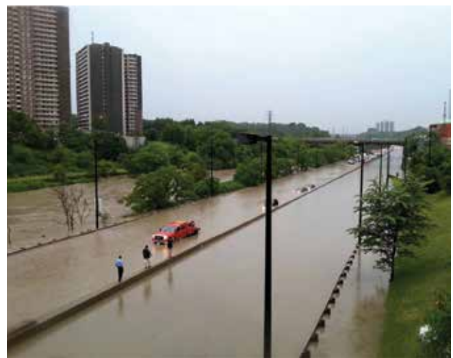
Photo credit: Toronto Hydro.
