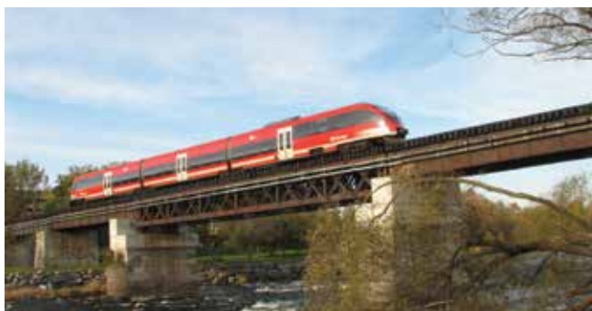
Ottawa's O-Train light rail transit (LRT) crossing the Rideau River. The Stage 2 extension is one of the projects jointly funded by federal and provincial infrastructure funds.
