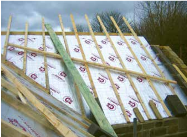
A home renovation where insulation was added to the envelope.
