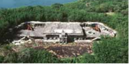
Battery Cheney, a gun emplacement on Corregidor, part of the island's powerful defences
