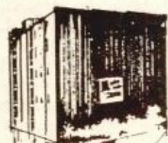
HOOSAC STORES - Possible demolition, adaptive use or curatorial storage.
