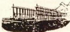
MARINE RAILWAY - Unfeasible to preserve. It will be documented and dismantled.
