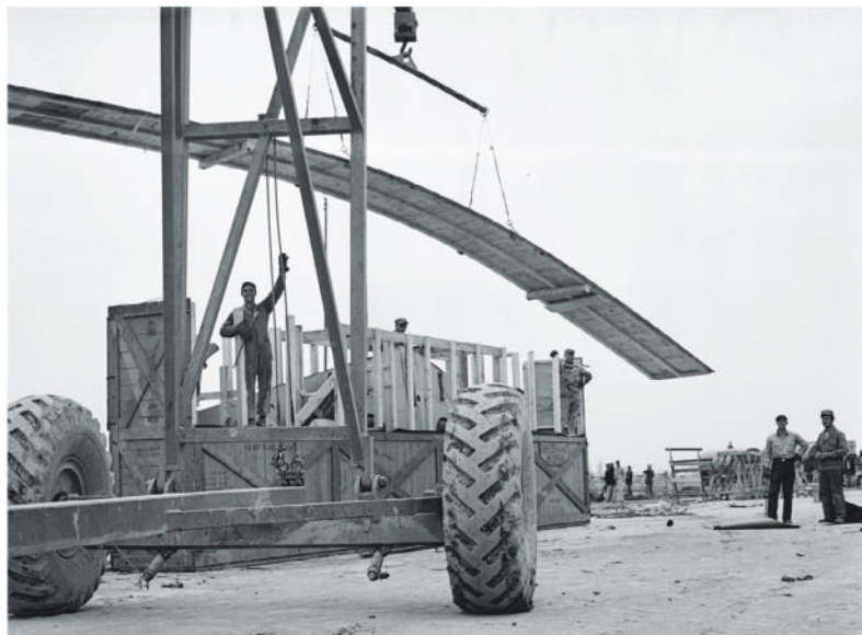
At Abadan, Persian Gulf Command crews broke open acres of crates containing aircraft components and transformed them into thousands of American-made fighters and light bombers flown to the Soviet Union through Iranian air space.
