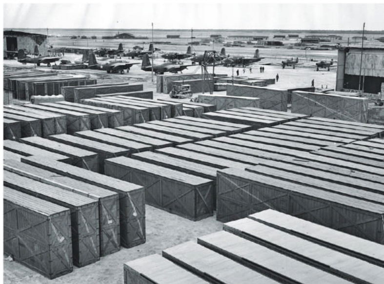
At Abadan, Persian Gulf Command crews broke open acres of crates containing aircraft components and transformed them into thousands of American-made fighters and light bombers flown to the Soviet Union through Iranian air space.
