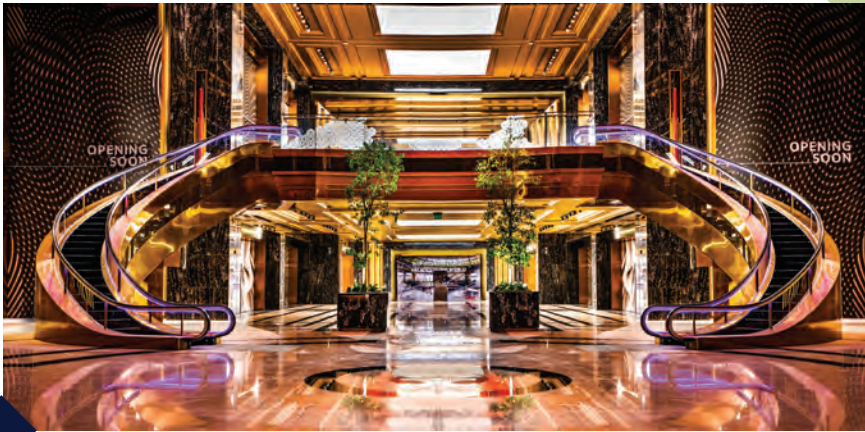
The curved outer sheathing for the spiral escalators has a combination of gold-colored stainless steel with etching designs, and the sandwiched soffit glass with bronze mirror has gold-colored mesh within.
