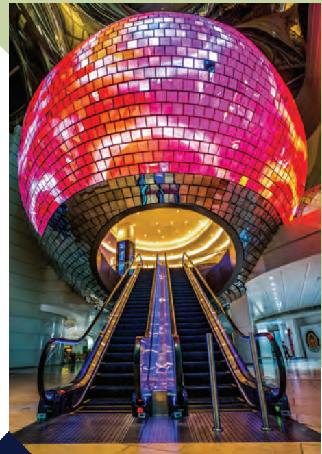
The curved outer sheathing for the spiral escalators has a combination of gold-colored stainless steel with etching designs, and the sandwiched soffit glass with bronze mirror has gold-colored mesh within.
