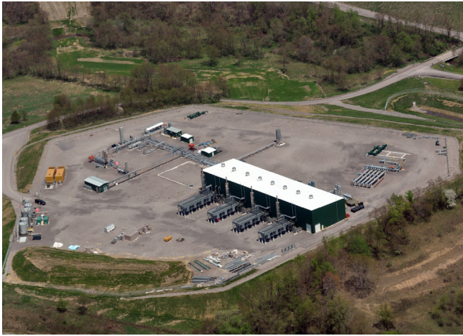
Trilith Compressor Station by Robert Donnan
