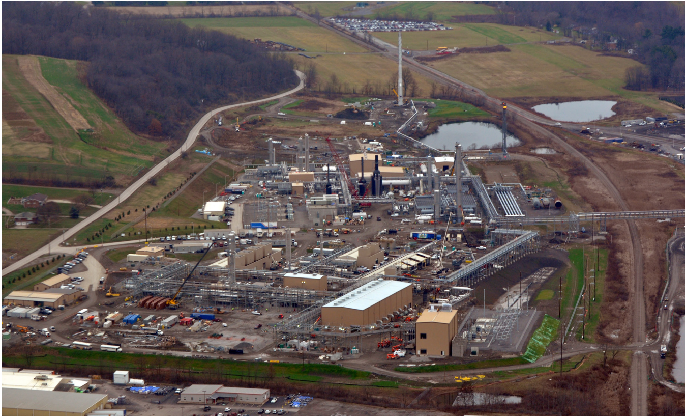
Bluestone Gas Processing Plant by Robert Donnan
