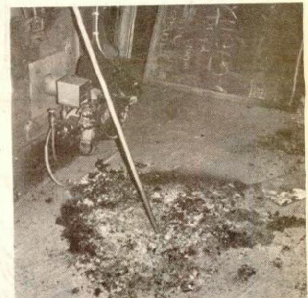
THE FIRE set adjacent to the furnace in the basement of the Old Kent School was, according to fire officials, made so as to appear accidental in origin. (photo by Kathy Giordano)
