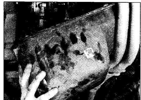
13.3 Removing the sump
