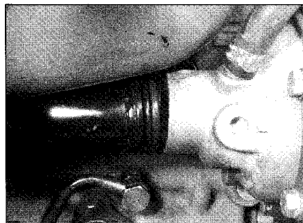
10.18b Removing the metal coolant return pipe from the water pump
