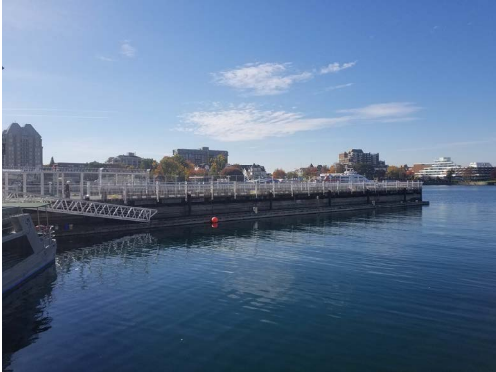
Photo 3 –Existing Ship Point wharf, north side
