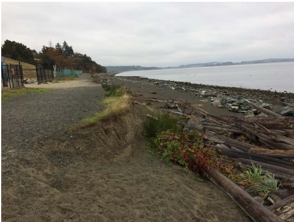
Photo 2 - Existing beach at proposed Royal Bay terminal site, looking north.
