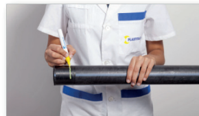
Mark the insertion depth.
