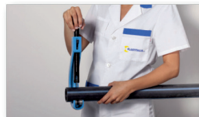
Cut the pipe with the pipe cutter.
