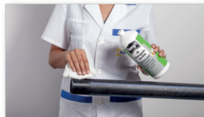
Clean the surfaces with a suitable detergent.
