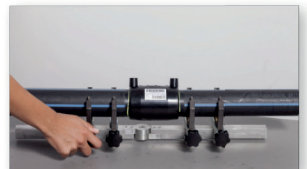
Clamps pipe and align it.
