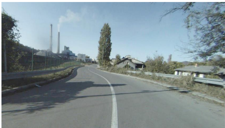
Figure 48. access street to the southern part of the complex (left - ashtray and heating plant)
