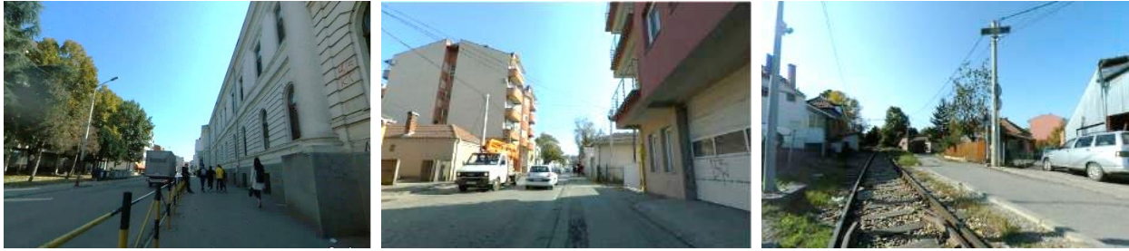
Figure 39. Kosovska Street in the area of the Mechanical-Engineering School; Figure 40. Constructed structure in Kosovska Street; Figure 41. The route of the industrial railway through a part of the residential zone;
