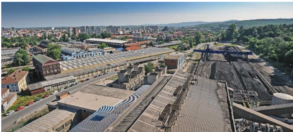
Figure 42. Panoramic view of the complex from the south side of the complex - view of the ash dump - part of zone 3.2 and part of the heating plant - zone 4.2 (close-up)
