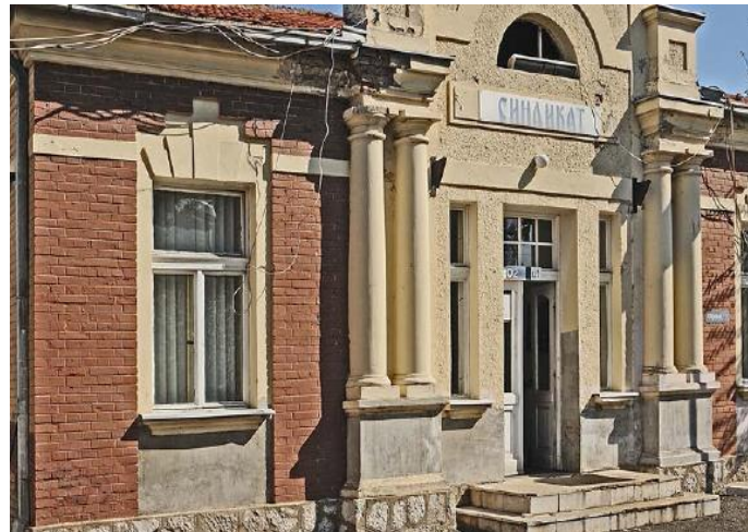
Figure 77. Old Ambulatory Care Building
