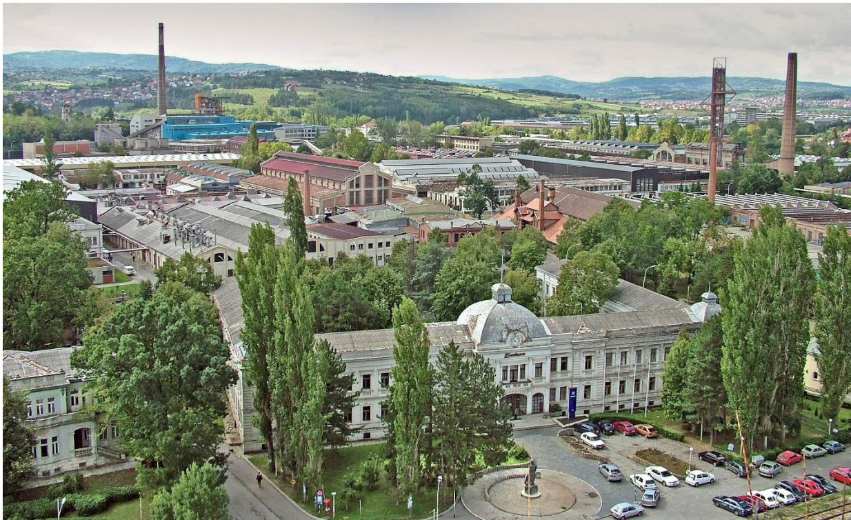
Figure 53. Panorama of the complex (foreground - square in front of the administrative building with the monument "Livac")
