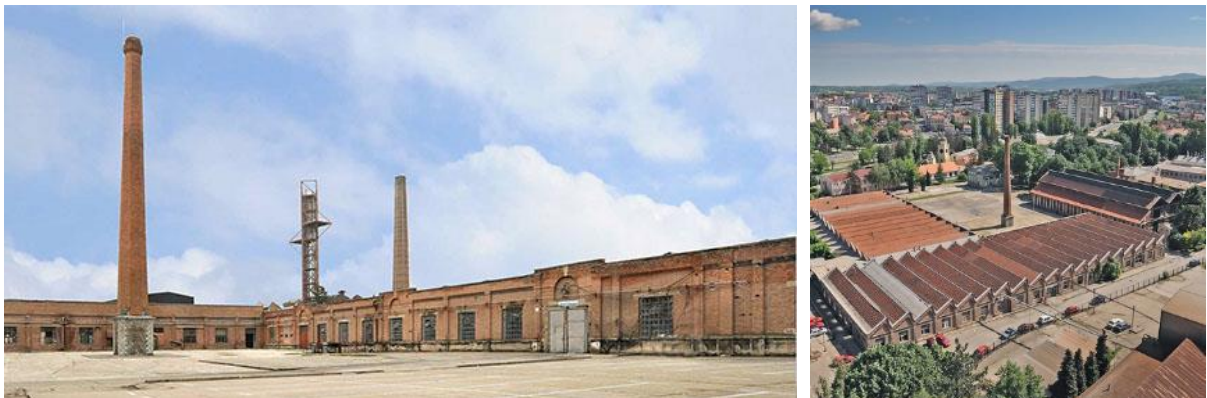
Figure 64., 65. u 66. Mechanical/machine shop
