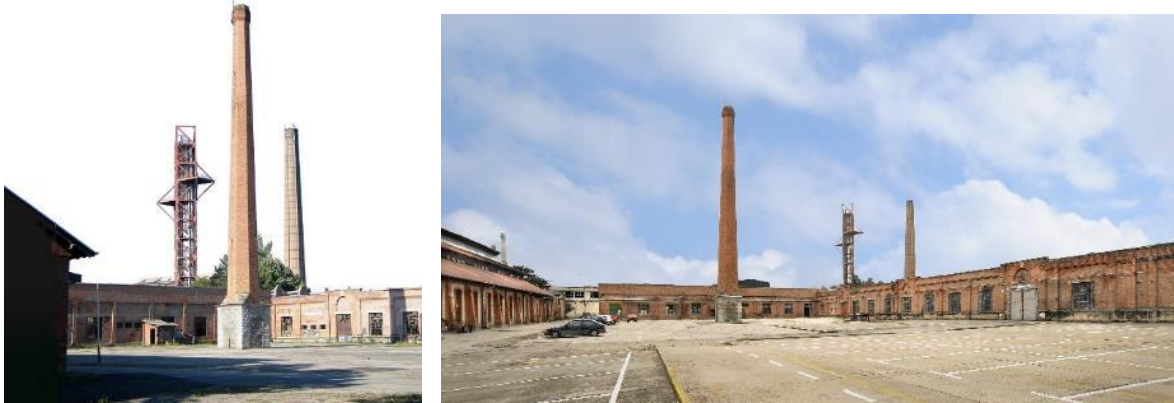
Figure 62. Old Tall Chimney
