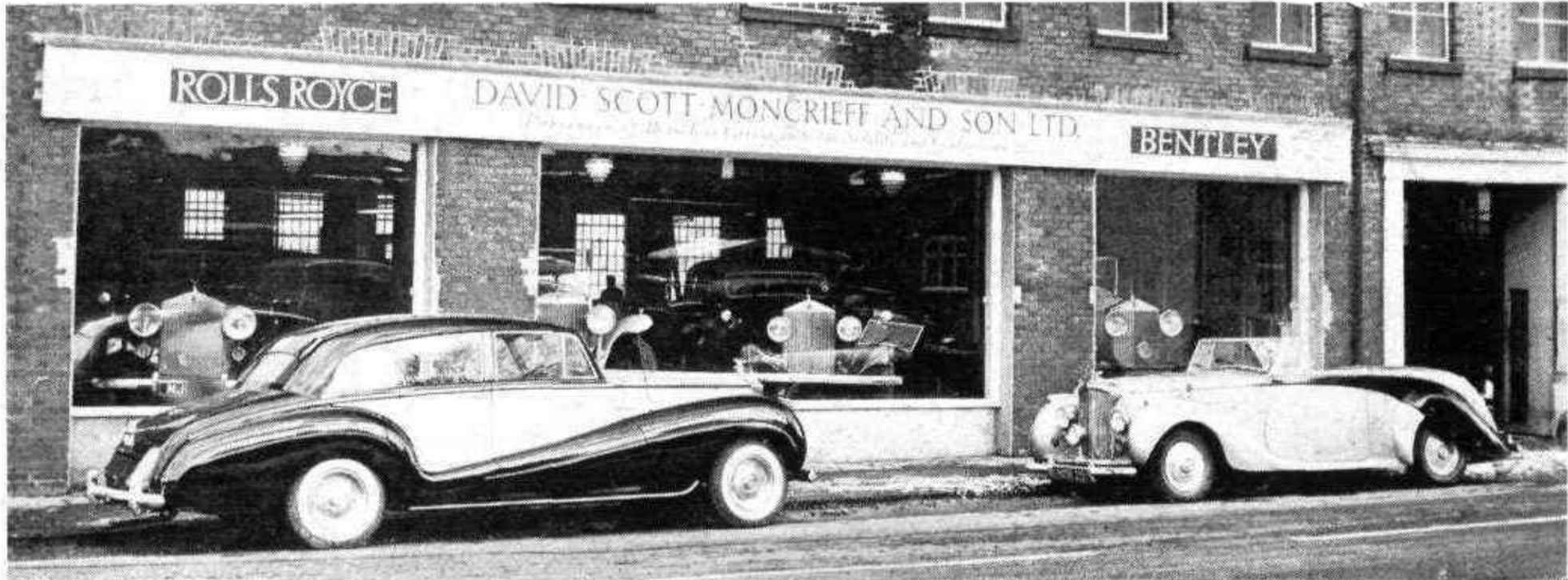
Showrooms at 2 Macclesfield Road, Leek, Staffordshire
