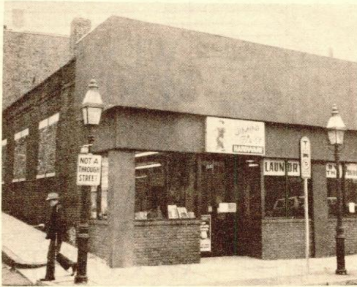
JIMINI FIX'IT Hardware Store on 251 Main Street is one of the most recent additions to the Charlestown business community.
