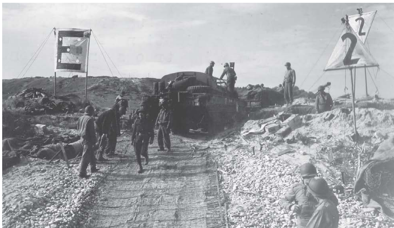
Exit E-1 between WN 64 and 65 looking inland. NARA
