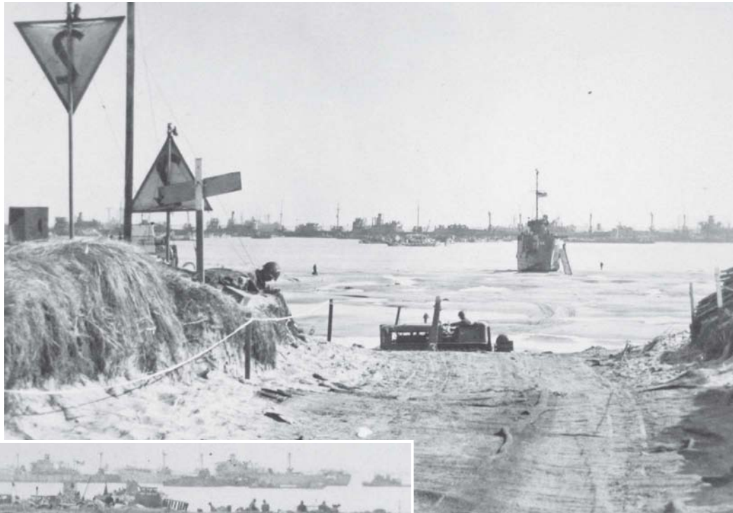
Below: The work at improving the exits at Exit E-1 went on for some time. This photo of a D7 bulldozer improving the road was taken 15 June. NARA
