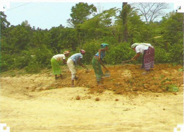
SHG women repairing the village road
