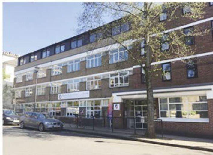
St Edmund's Terrace. School's front facade
