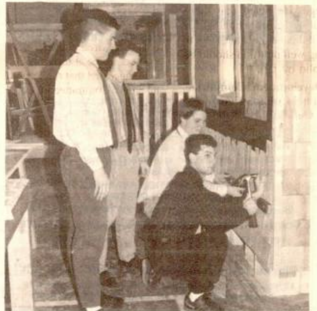
PUTTING THE FINISHING TOUCHES on the house constructed on the sixth floor of Don Bosco Technical High School in Boston by students of the Building Technology department are: standing (l. to r.) Stephen E. Power of 9 Hill St. and James Burke of 26 Cross St., both of Charlestown and kneeling (l. to r.) Joseph C. Murphy of Brighton and Roberto P. Barletta of Allston.
