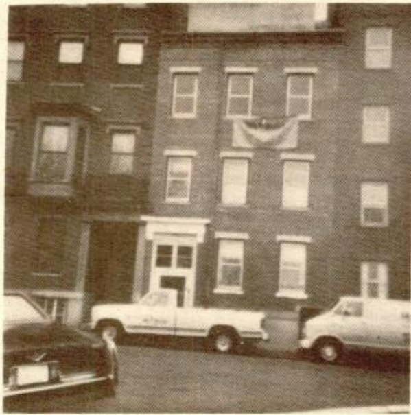
THE HOME of Jim and Patti Lyons on the Training Field is being renovated by Mr. Build LRE Construction Co.
