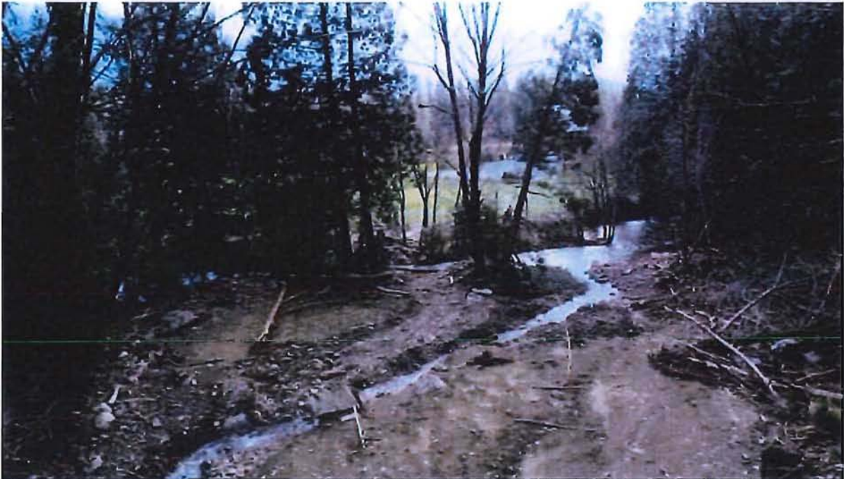
Figure A-7: Ground level view of newly deposited debris flow with minor stream cutting through. Site 02C
