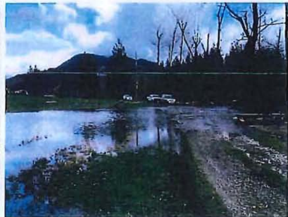
Figure 3-4: Road washout caused by landslide redirecting flows from Hicks Creek. Site 02D.
