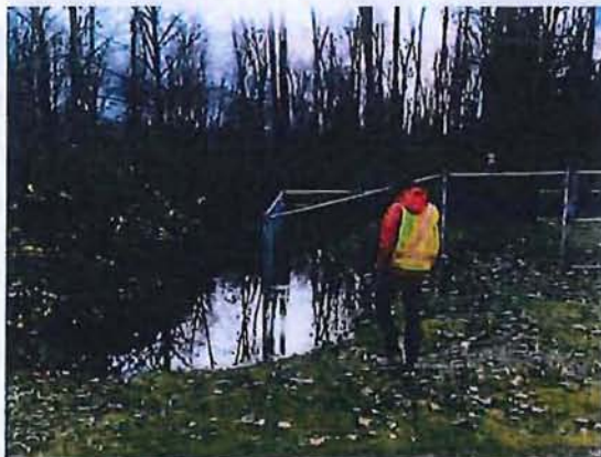
Figure 3-9: Tetra Tech staff inspecting ponding near sewage lift station on Strawberry Island
