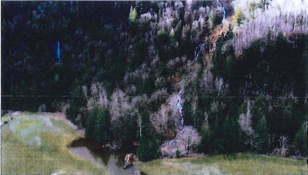
Figure A-5: Aerial Image Northwest Landslide and Channel Blockage. Site 02C.
