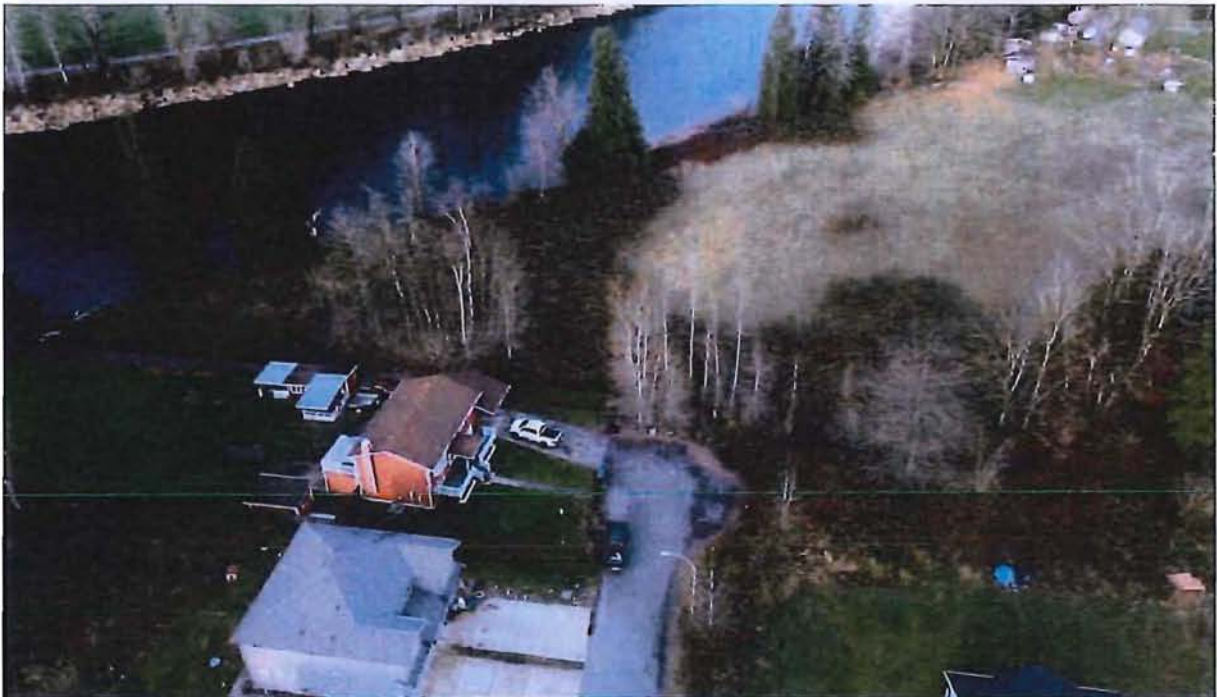
Figure A-19: Aerial view of Strawberry Island development and shared bank with Maria Slough
