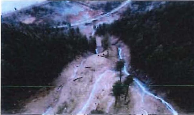
Figure 3-7: Landslide near Highway 7 looking downslope
