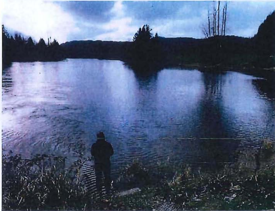
Figure A-21: Surcharged Culvert servicing private District of Kent Driveways. Site 05D
