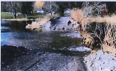
Figure 3-11: Deconstructed Private driveway.
