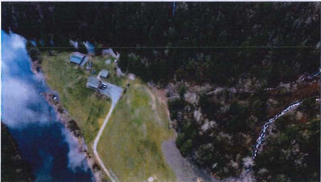
Figure A-8: Aerial Image Northwest Landslide and Channel Blockage. Site 02C/02D
