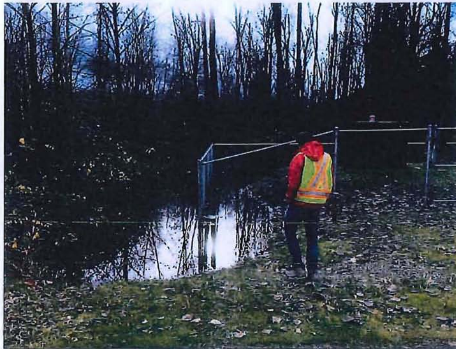
Figure A-17: Tetra Tech staff inspecting ponding water near developments sewage lift station
