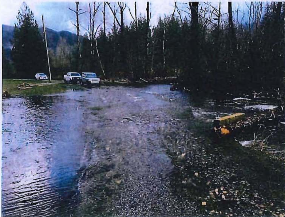
Figure A-10: Road washout due to channel blockage. Site 02D
