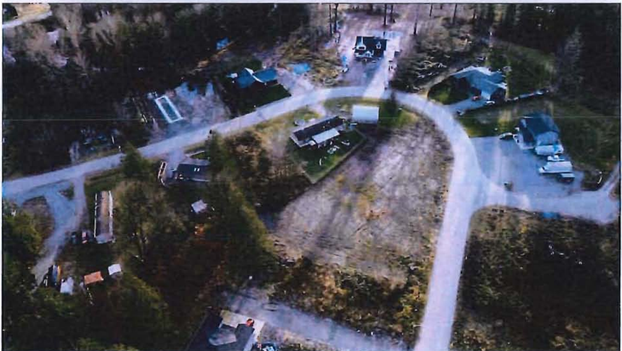
Figure A-20: Aerial view of Development. Ponding can be seen on several sights at top of photo.
