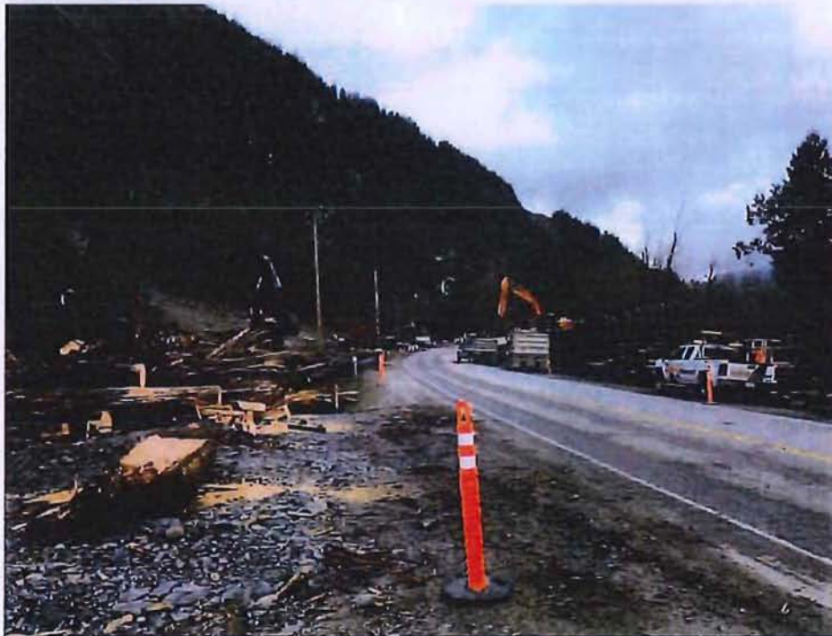
Figure A-16: Progress of landslide remediation at time of site visit
