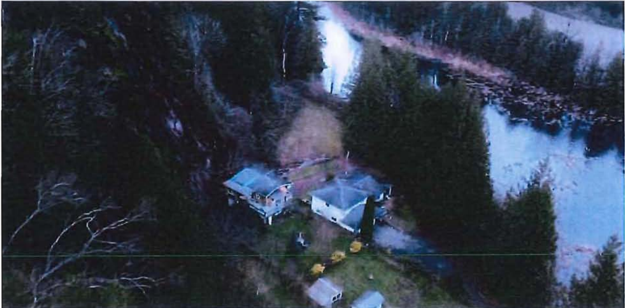
Figure A-11: Landslide and debris near District of Kent private property. Site 02B
