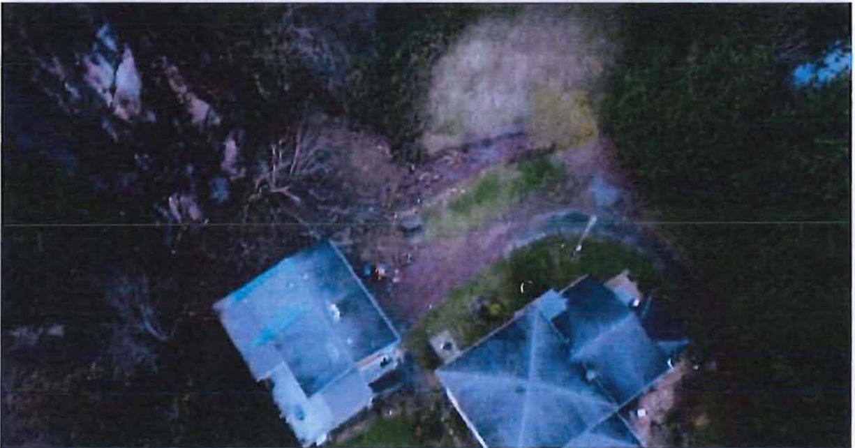
Figure A-12: Landslide and debris near District of Kent private property. Site 02B
